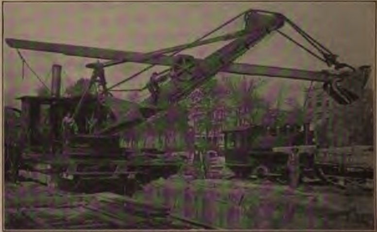
Steam Shovel on Sewer Trench Excavation.
